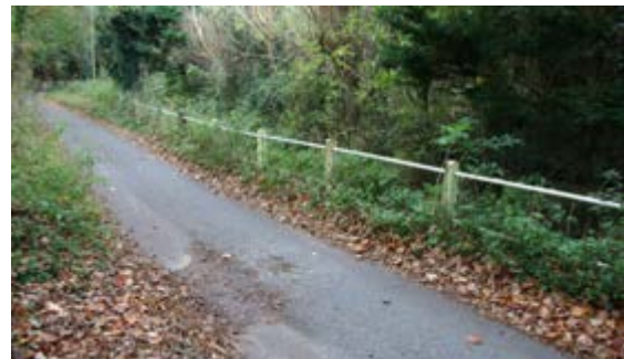
Concrete posts and iron guard rail on Tiggins Lane, providing a safety barrier between the road and stream
